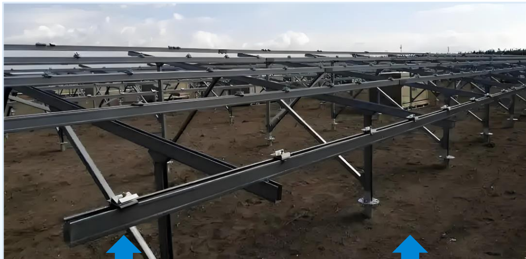
Figure 1. PV module installed with bolt fitting method.
