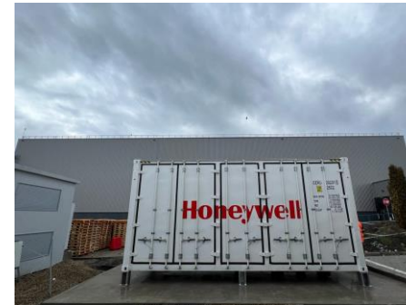
BESS 1.2MW/1.6MWh
