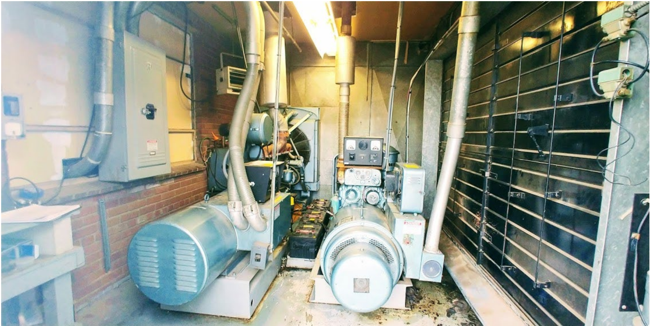
WWII era generator set backing up the hospital
