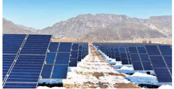
Global Largest Ground-mounted Power Plant Using Shingled-cell Modules. Henan, China | 5MW
