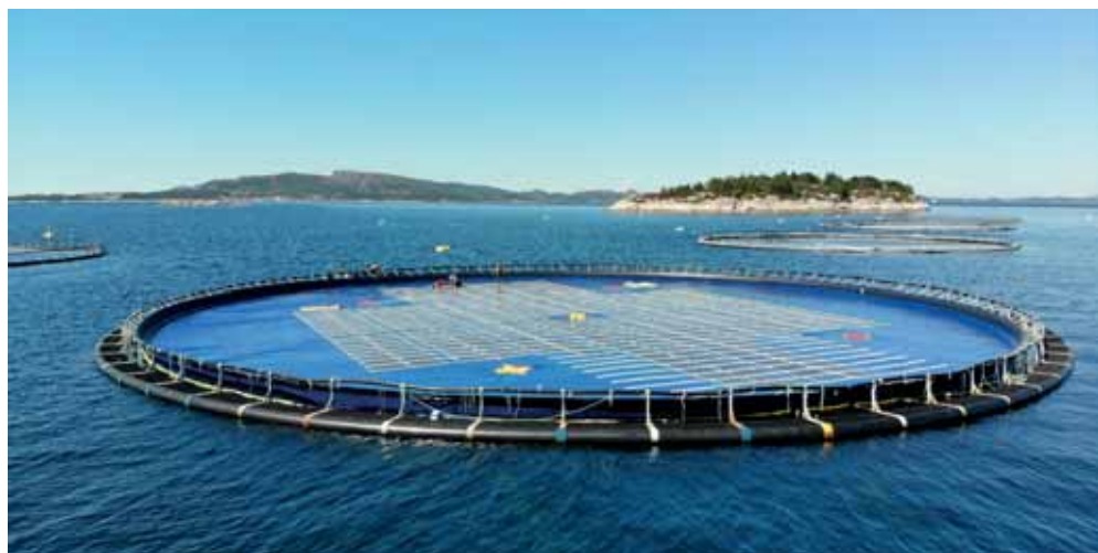
Figure 5. Off-grid installation powering a large fish farm at the west coast of Norway
