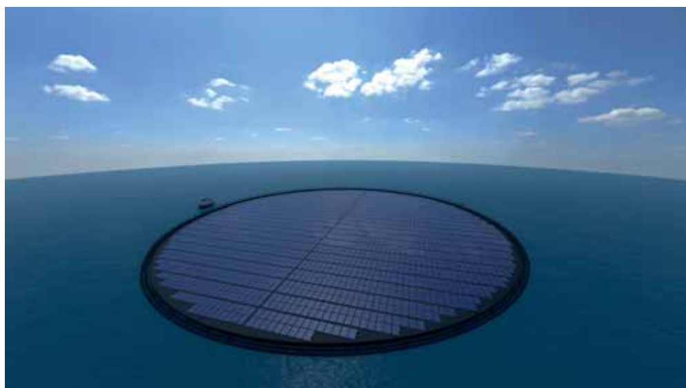
Figure 6. Illustration of a 1MW floater with a diameter of 100 meters
