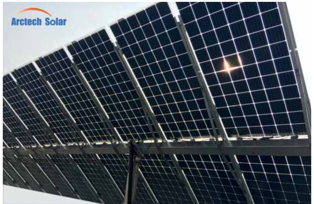
Figure 3. Independent horizontal single-axis tracker from Arctech Solar, designed for bifacial modules [145]. The modules are fixed using aluminium elements at the module edges, overlapping with the long purlins to avoid covering the back of the bifacial modules. Junction boxes at the module edges in such a system, as shown, can be integrated without shading caused by cables.
