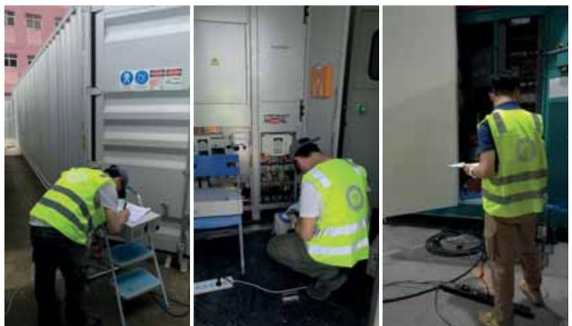
Safety tests on containerized Battery ESS
