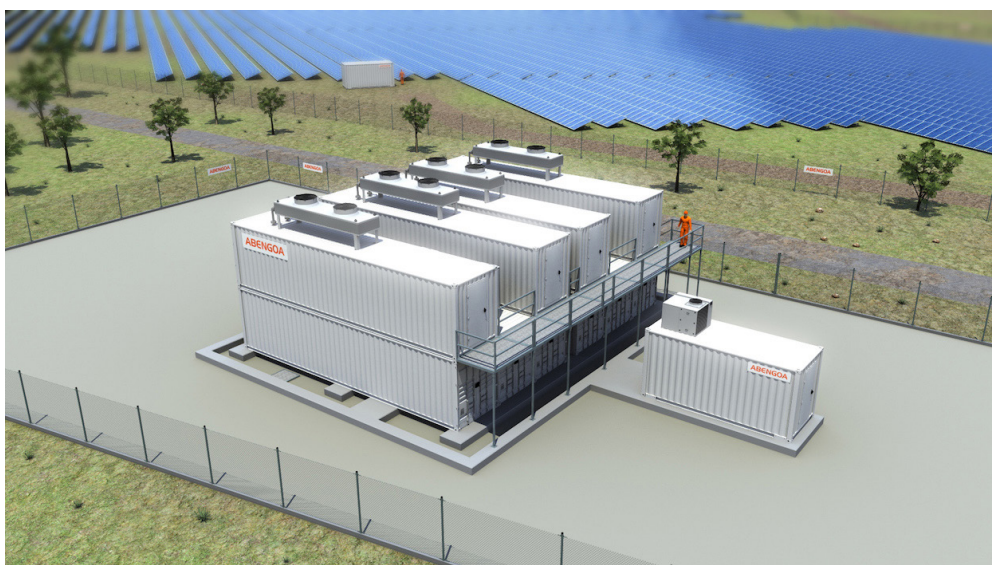
Bushveld Energy contracted Abengoa to deploy a VRFB system for a solar microgrid at its Vametco production site.
